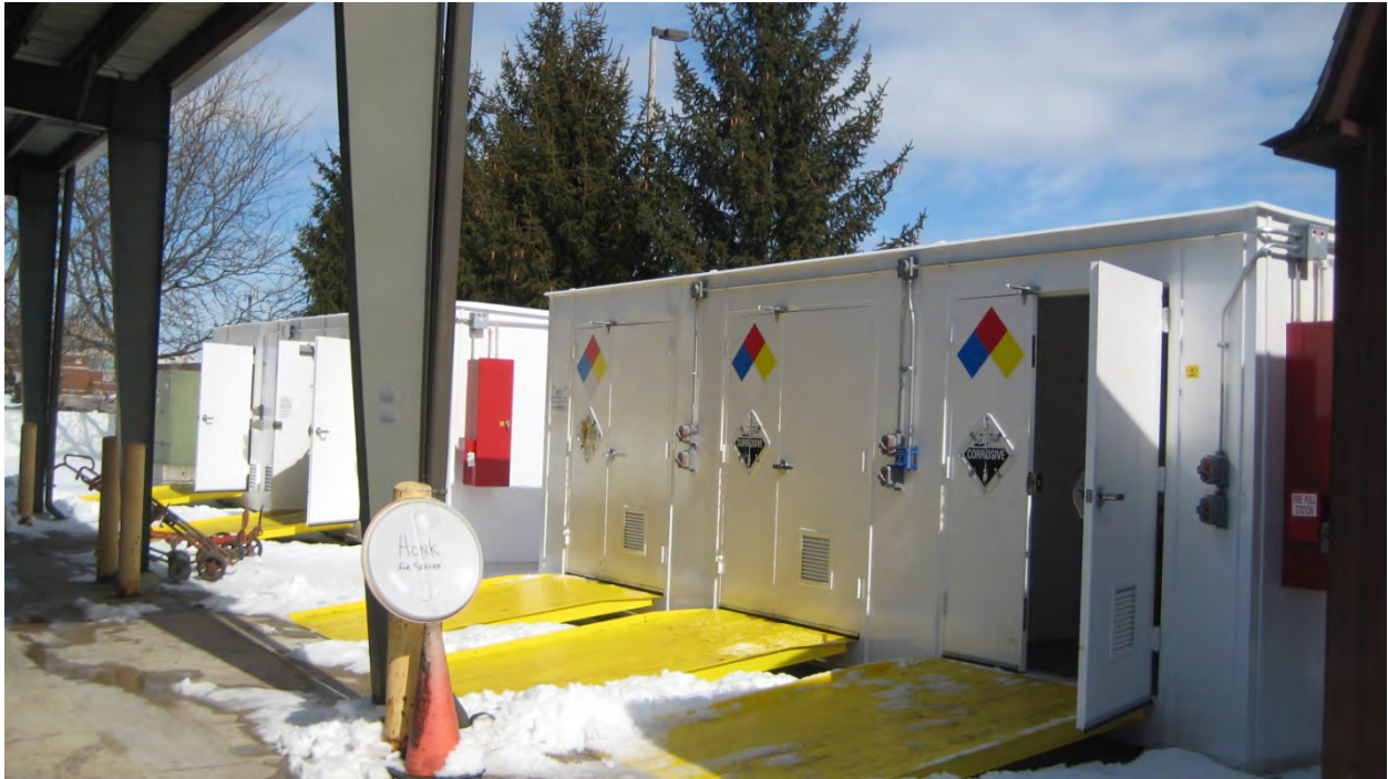
Figure 3-5. Secured Prefabricated Hazardous Material Storage Units at Naperville Facility.
