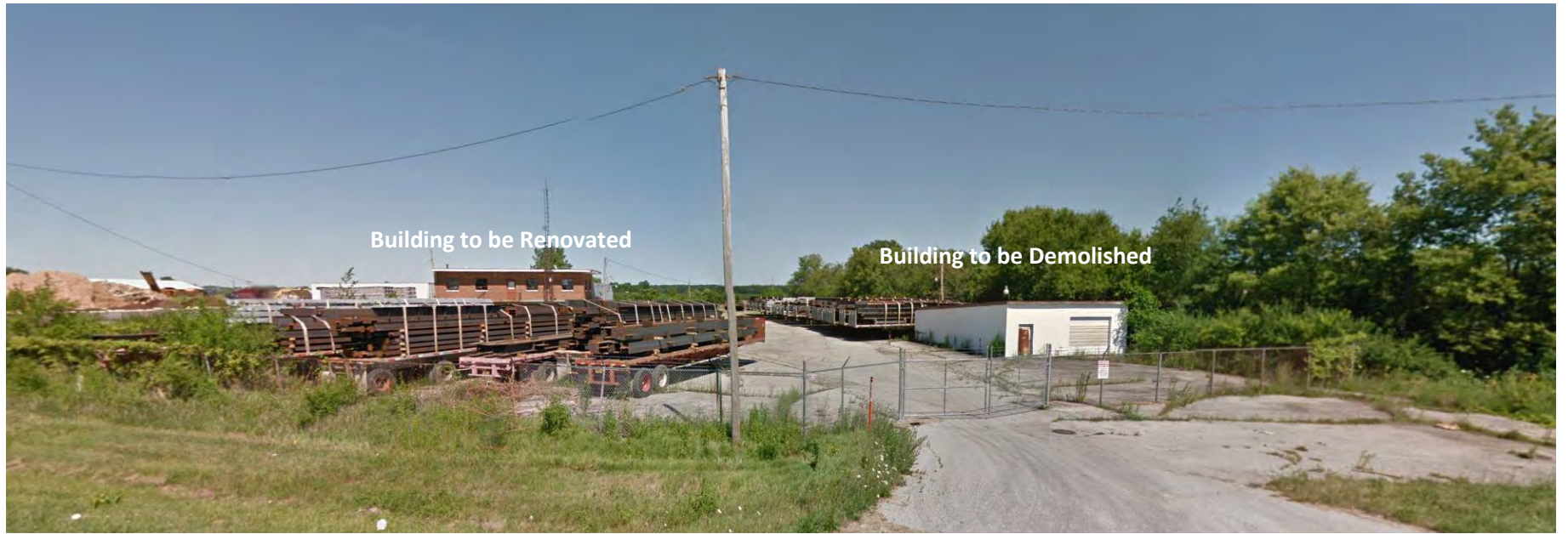
Exhibit D: Site Photo, Looking East
