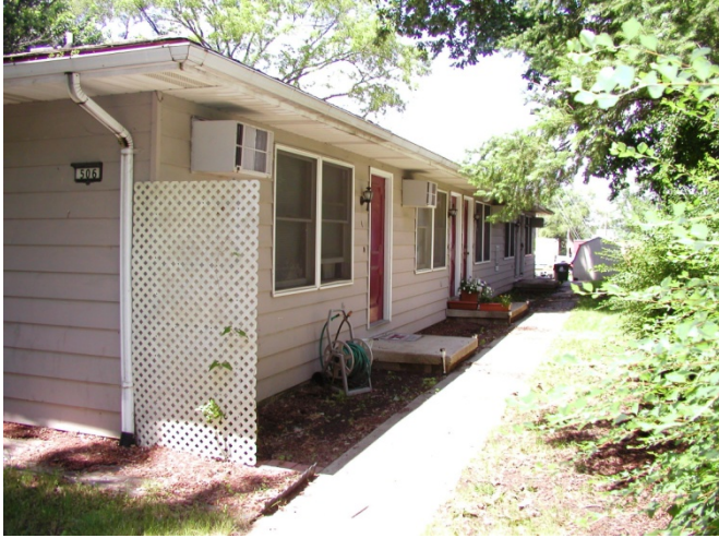
Figure 3. 506 East Elm Street – east elevation
