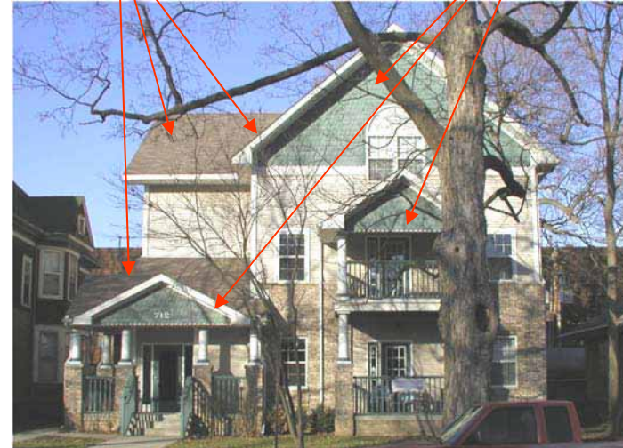
This new apartment building, outside of the corridor, makes use of changes in the wall plane, building height, and roofline
