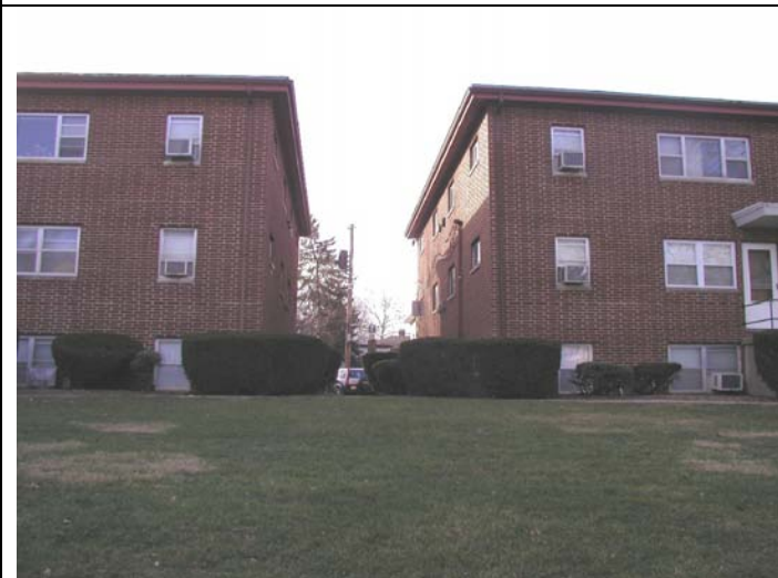
View south from Illinois Street sidewalk at space between buildings.
