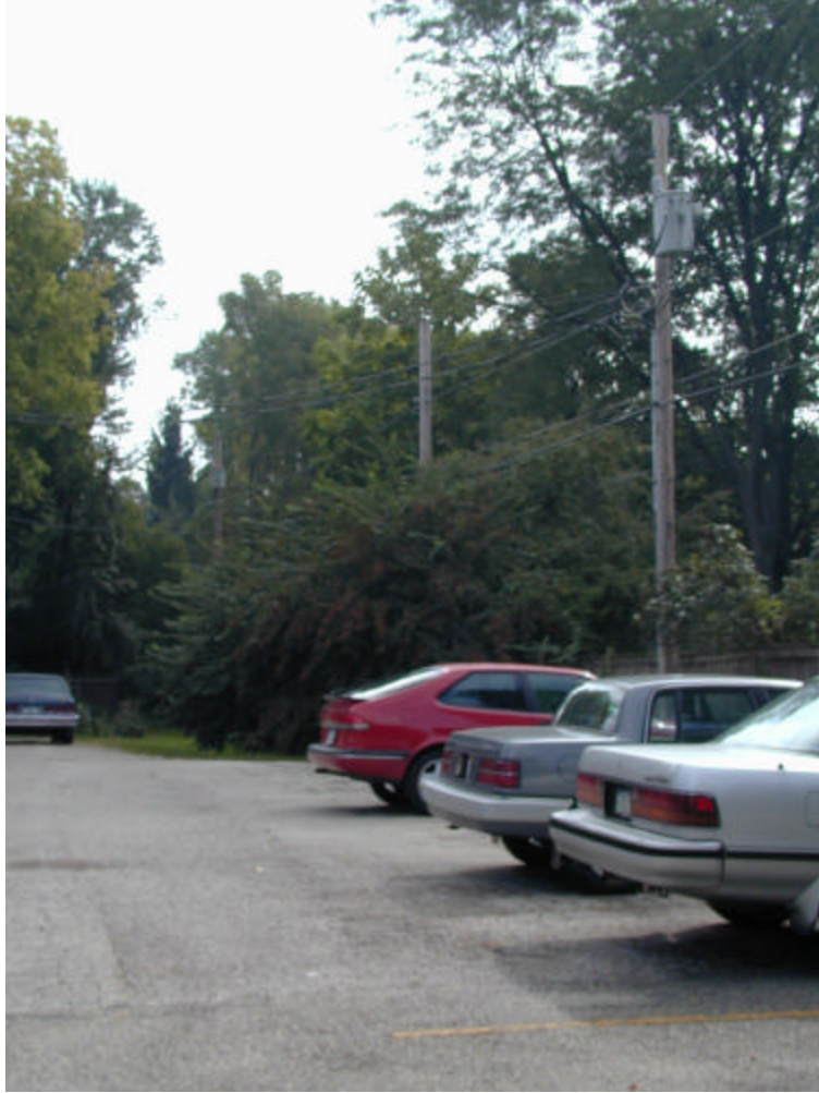
Attachment #2: Photograph of existing overhead utilities.
