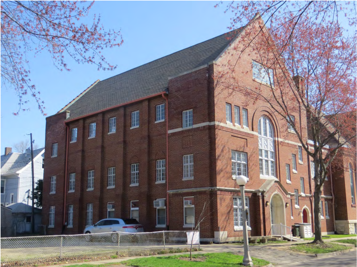
Classroom Addition on west side:
