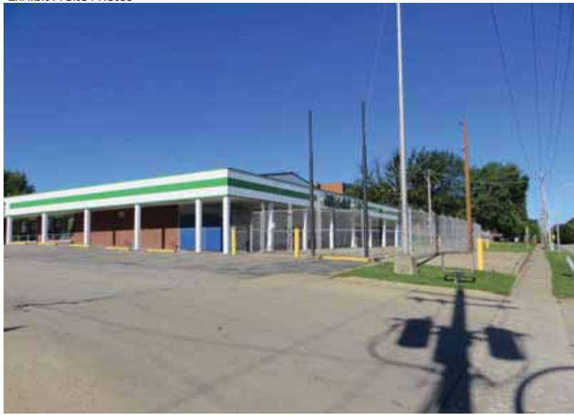
Looking east, from sidewalk
