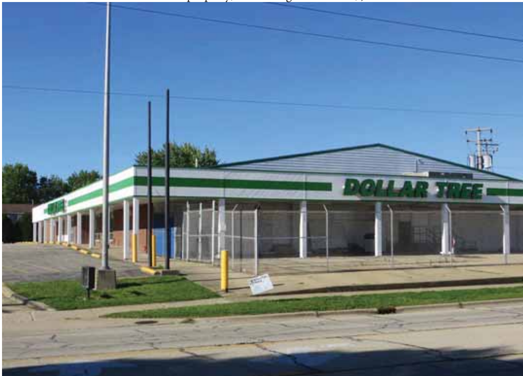
Front of property, looking south
