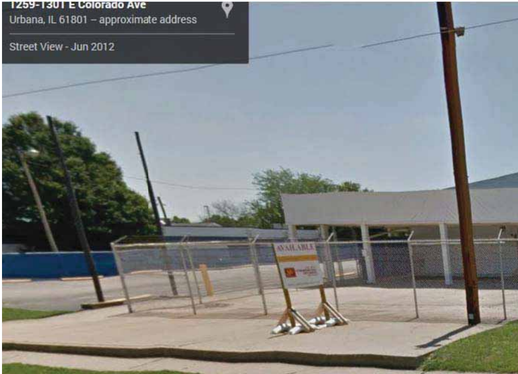
Front of property, from Google Streetview, June 2012
