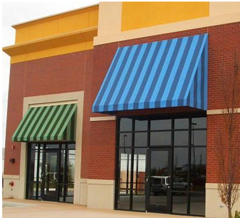
Figure 1: Much like the shade awnings shown above, the proposed shade awning for the subject property would require no support columns.
