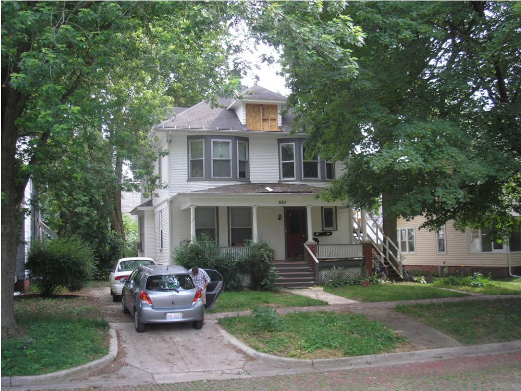
Figure 1. Existing House, front façade
