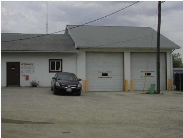
Tatman's Towing, east portion of building along Perkins Rd
