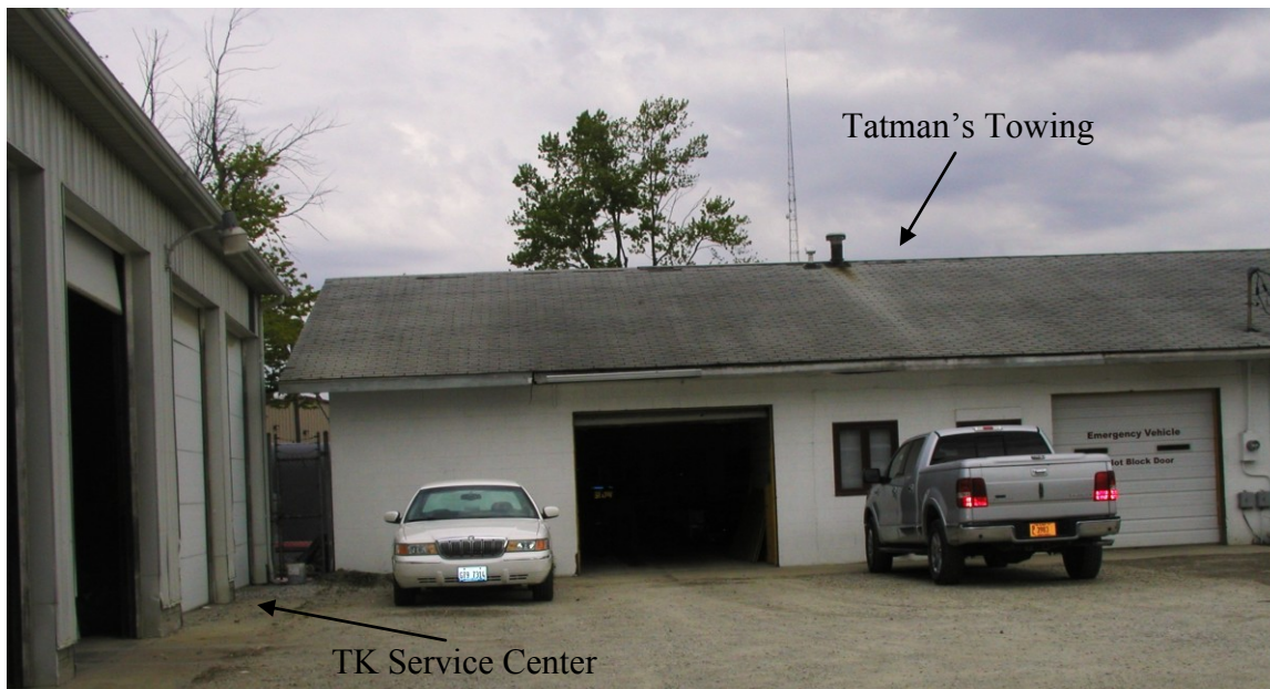
Overhead doors on the TK Service Center and Tatman's Towing buildings
