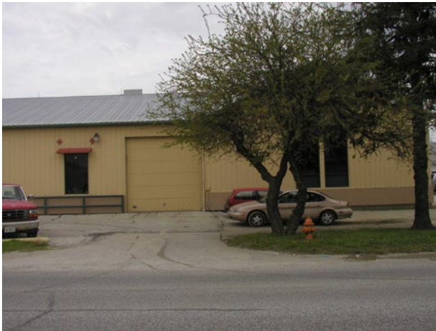
TK Service Center, mid-section of building along Perkins Rd
