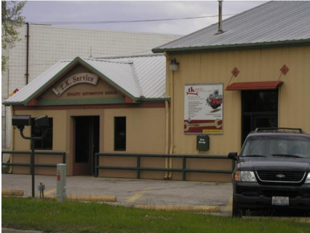
TK Service Center, west portion of building along Perkins Rd
