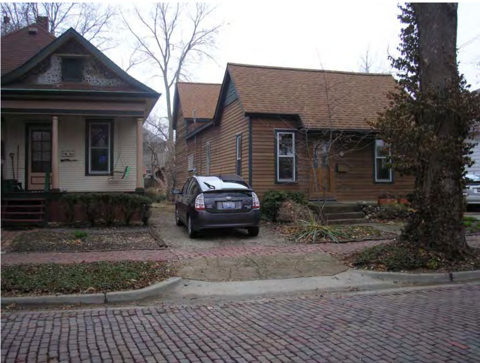
Figure 4. Existing House, west elevation – location of earlier addition
