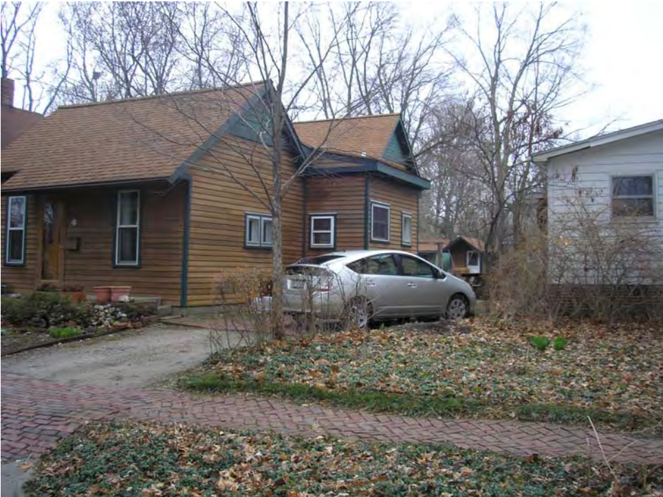
Figure 2. Existing House, east elevation
