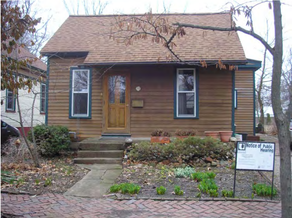
Figure 1. Existing House, front façade
