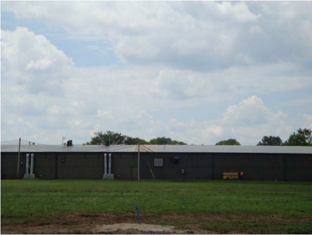
East elevation of property immediately west of subject parcel.
