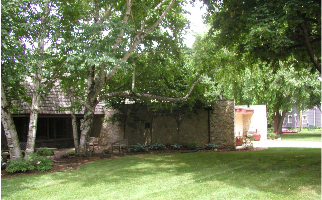
Figure 3: View of west side of parish center with sign.
