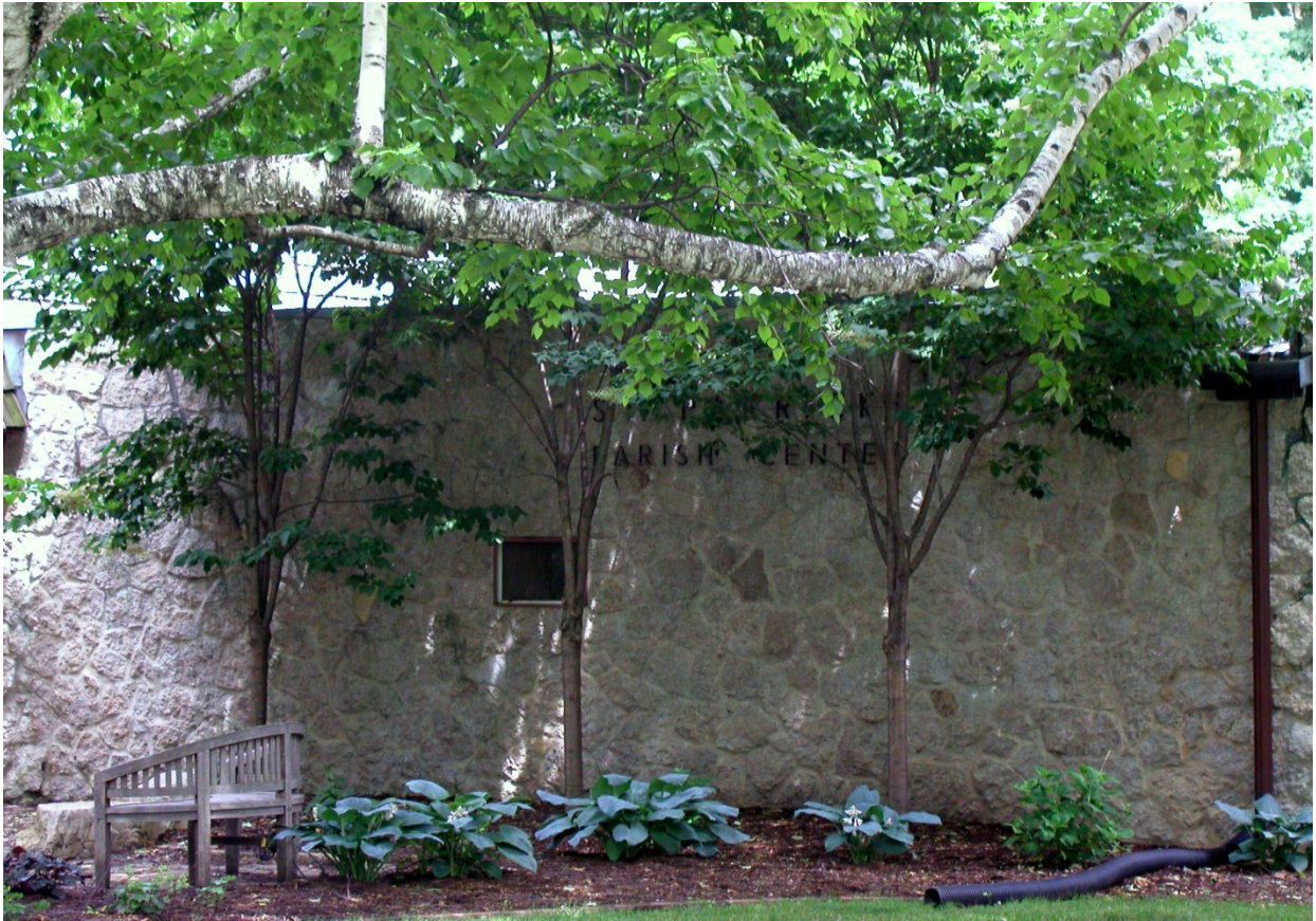
Figure 4: Close-up of parish center sign on west wall.
