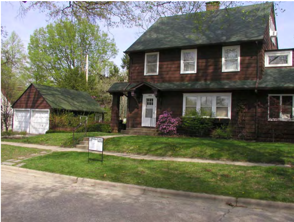
Figure 3. House and Garage, Orchard Street
