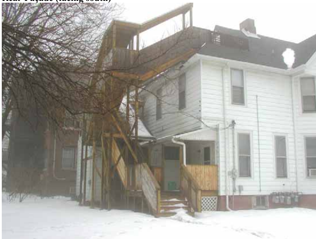
Rear Façade (facing south)
