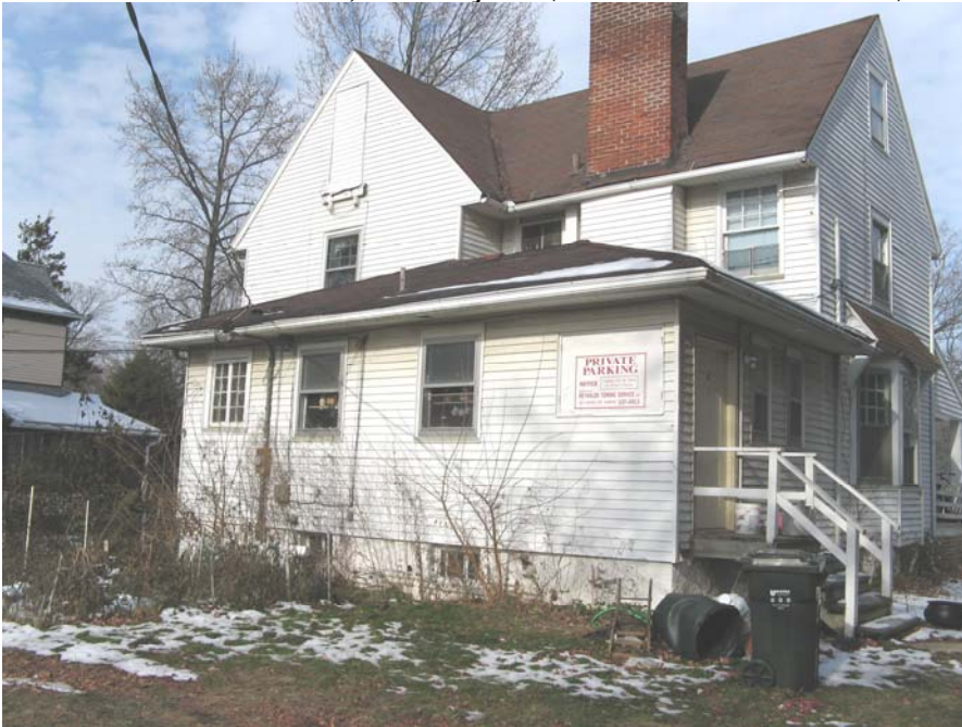
3. 605 W. Green Street, rear façade (south & east elevations)
