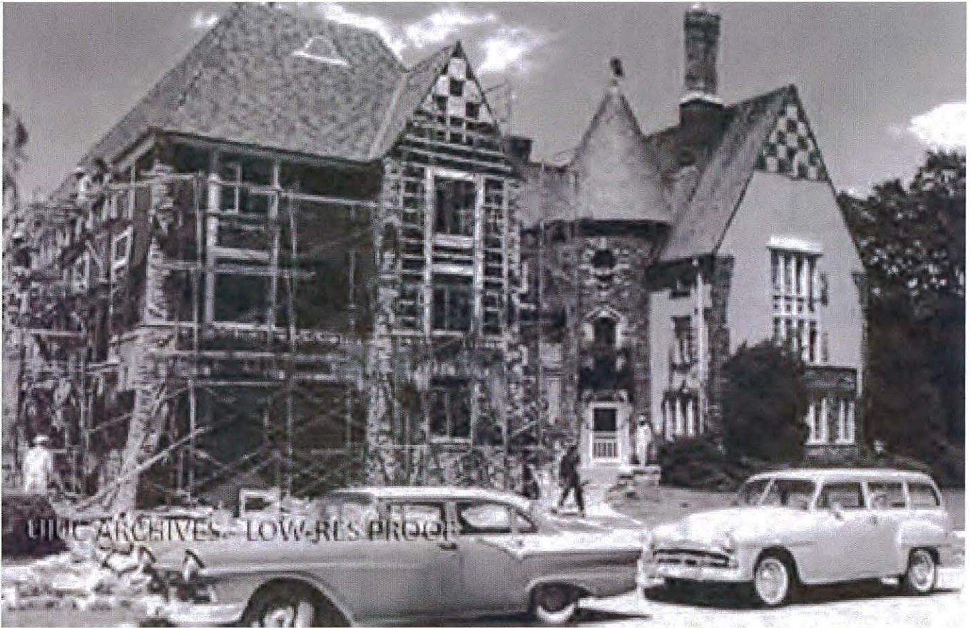
Zeta Tau Alpha House Addition Under Construction, 1962
