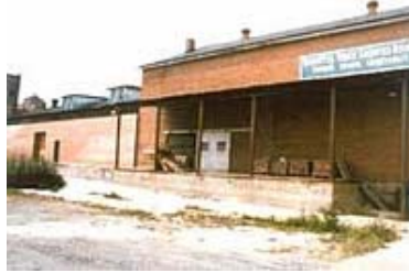
As part of a rehabilitation project, a late-19th century produce distribution center (top left) with a utilitarian loading dock (top right) was removed and replaced with a monumental entrance featuring massive formal columns (left). The new addition is incompatible with the simple, industrial character of the building. Photos: NPS files.
