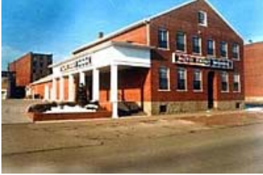
As part of a rehabilitation project, a late-19th century produce distribution center (top left) with a utilitarian loading dock (top right) was removed and replaced with a monumental entrance featuring massive formal columns (left). The new addition is incompatible with the simple, industrial character of the building. Photos: NPS files.
