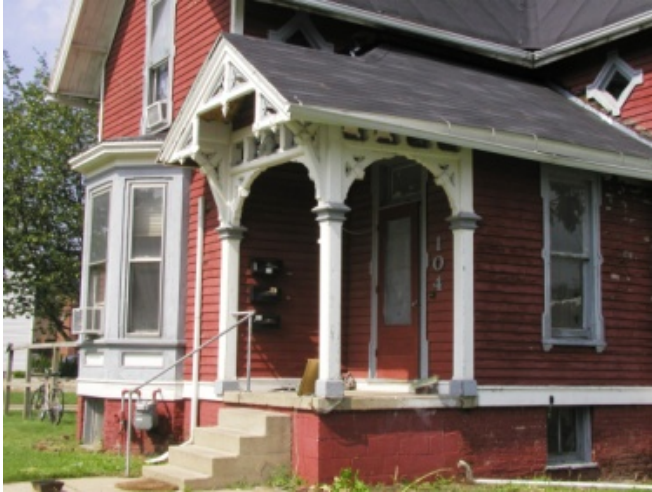
Halberstadt House, Front Façade, Existing
