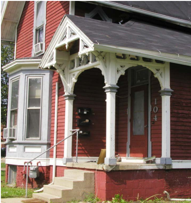
Close Up of Front Porch
