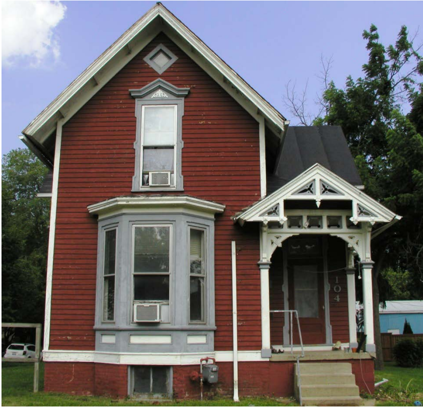
Halberstadt House, Front Façade
