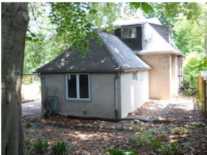
back of house (looking northeast)
