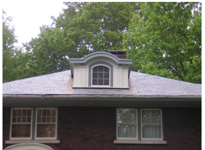
Dormer on front façade
