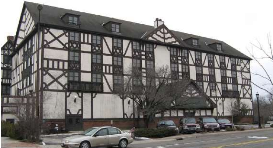
Nearly entirely 1980s addition
