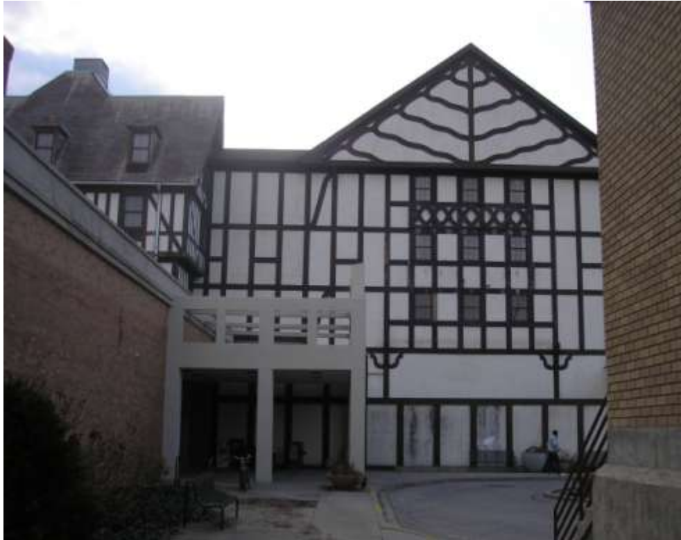
Windows in Urbana-Lincoln Hotel with views of proposed tower
