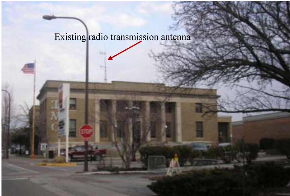
Front (west) façade, with existing roof-mounted radio transmission antenna visible
