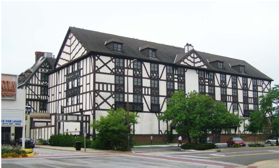
Conference Hall, North 1982 Addition
