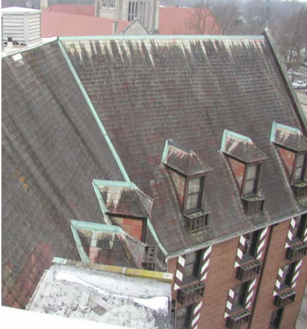
View of Transite shingle roof
