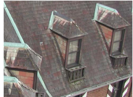
Close up of shingles on dormers
