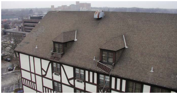
Close up of asphalt shingles on 1982 addition
