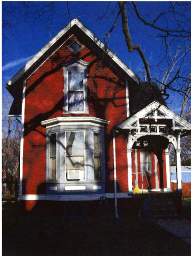
View of west elevation.
