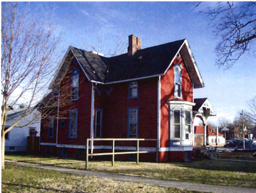
View of north and west elevations. View is towards the southeast.
