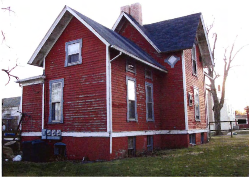
View of north and east elevations. The view is towards the southwest.
