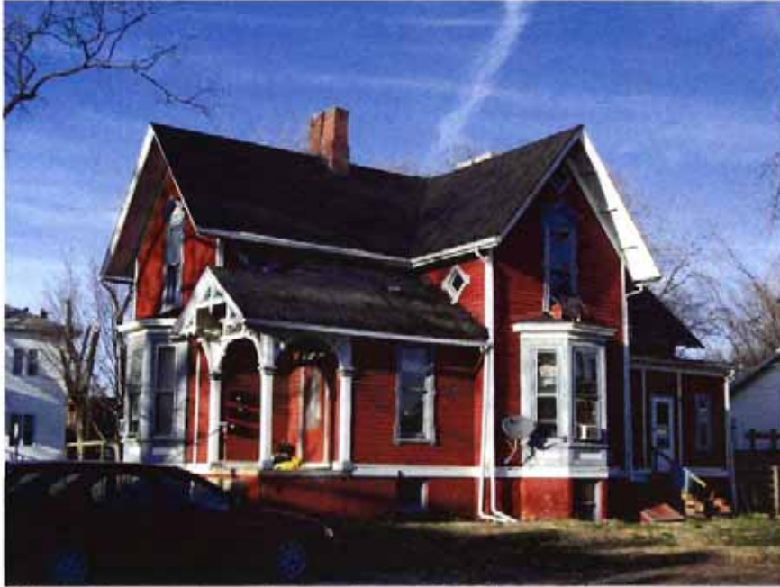
View of west and south elevations. View is towards the northeast.
