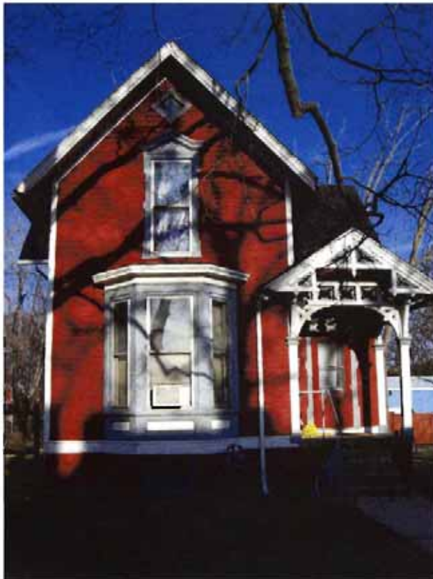
View of west elevation.
