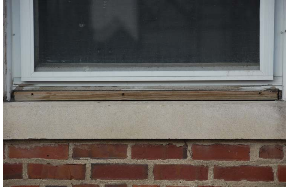
Bottom sill has been replaced with temporary board
