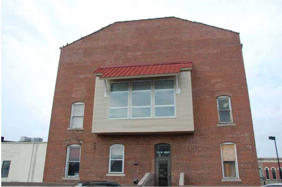
South elevation showing 5 windows proposed for replacement
