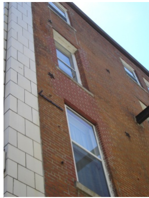
West (side) elevation, middle window
