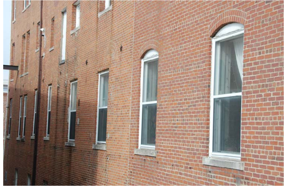
West elevation with window mix of half-moon tops and flat tops
