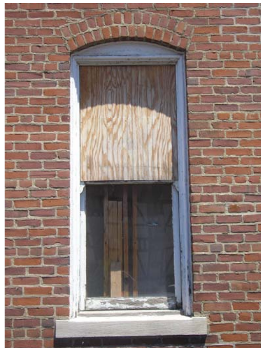
Lower right window, detail
