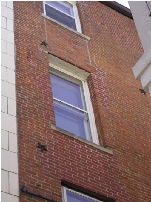
3 rd story window on west elevation, detail
