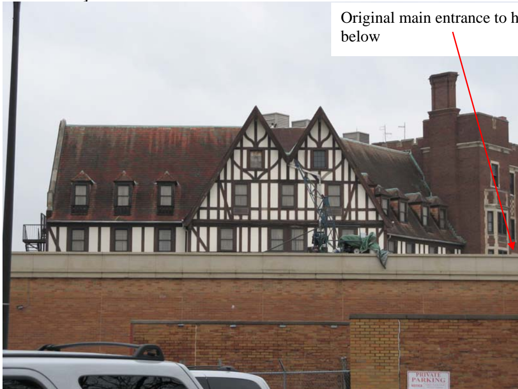
South façade, 1923 hotel, visible above 1964 Lincoln Square Mall addition
