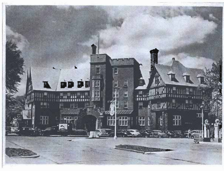
Early 20 th century views of the Urbana-Lincoln Hotel (southeast façade)
