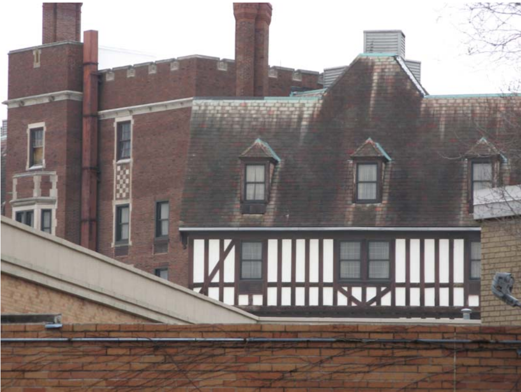
Close up of original 1923 building, east façade
