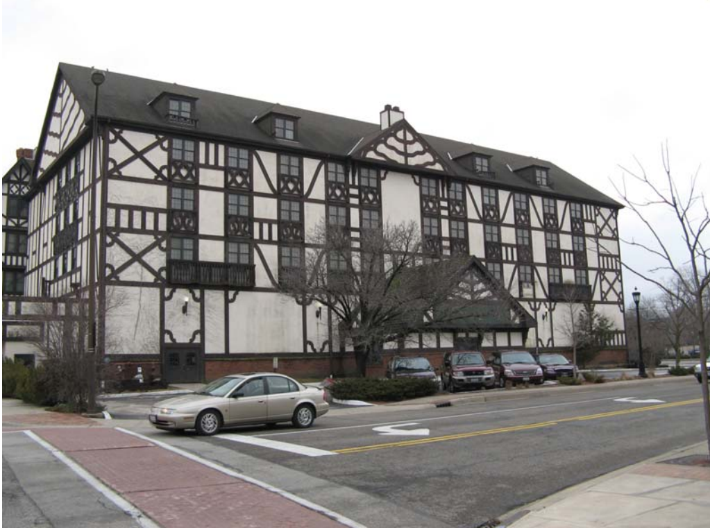
North façade, nearly entirely 1980s addition
