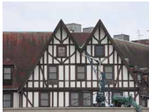
Another view of south facade
