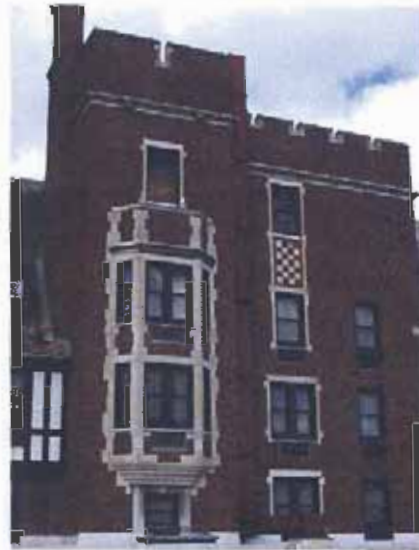
Detail, southeast facade
