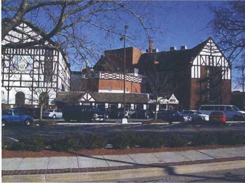
Current west entrance
