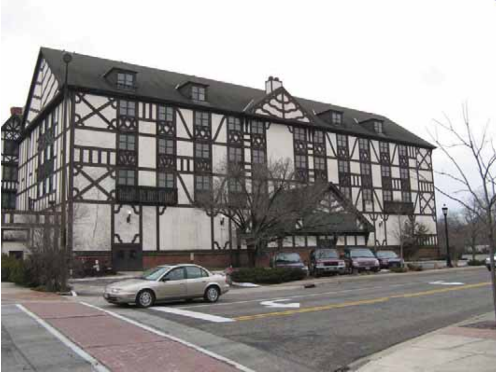
North façade, nearly entirely 1980s addition
