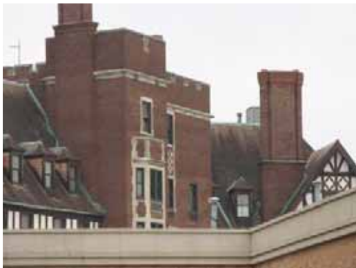
Another view of south façade
