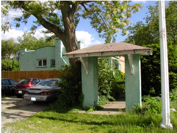
Courtyard Entrance Arch, looking south. 2006 Photo by Rich Cahill.
