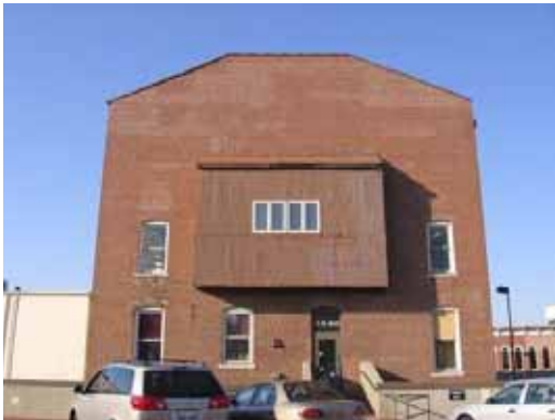
Rear (south) façade, 3 rd Floor extension. Photo taken from parking deck.
