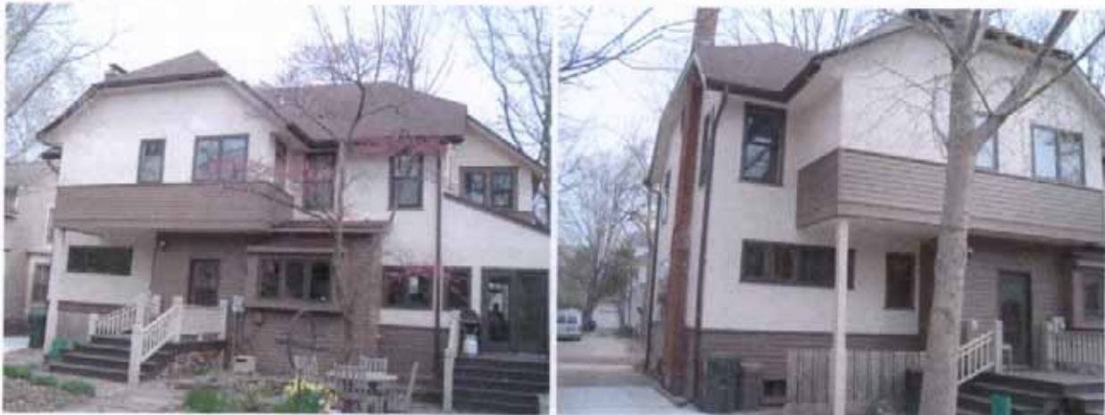
The current rear façade
