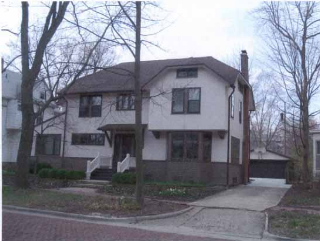
The north and west facades—taken looking south-southeast
