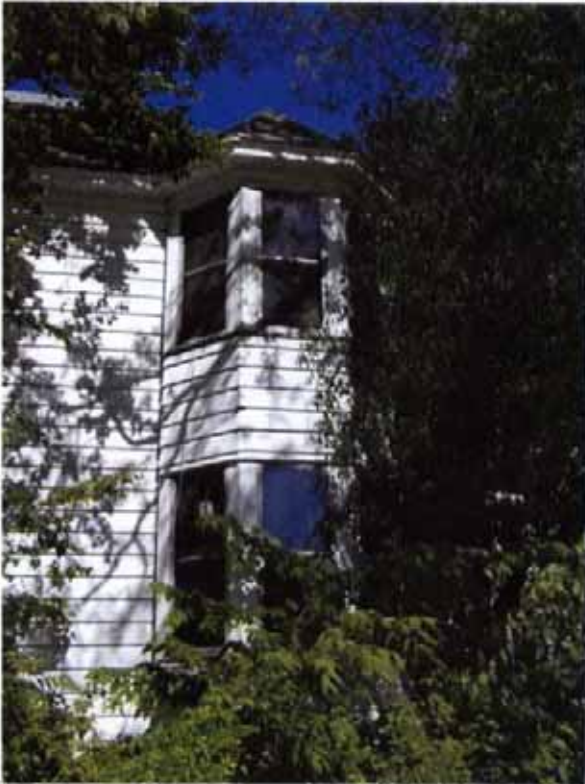
508 West Elm Street. Southwest corner tower.
