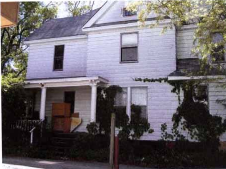
508 West Elm Street. East elevation.
