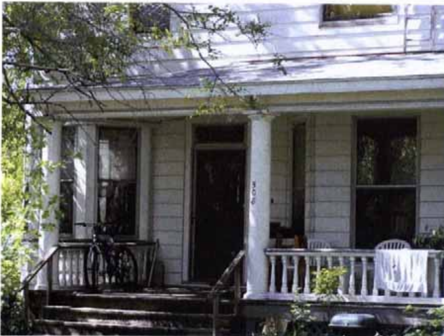
508 West Elm Street. South elevation, porch detail.
