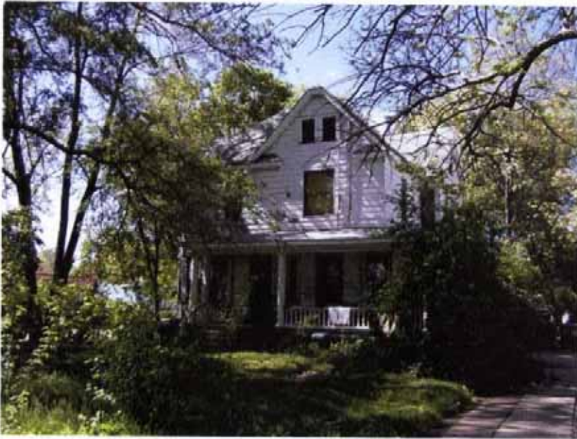
508 West Elm Street. South elevation
