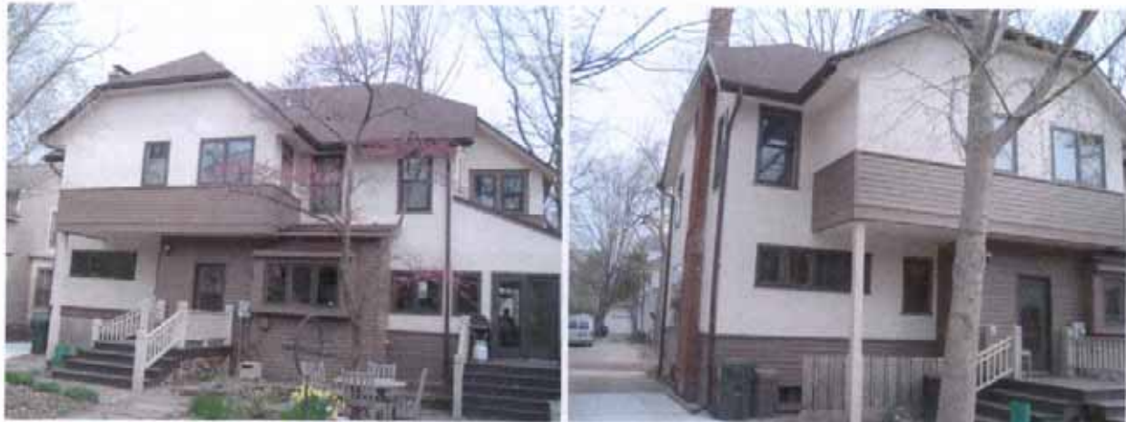
The current rear façade
