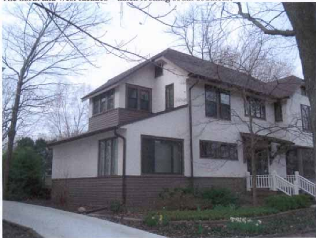
The east and north facades—taken looking southwest
