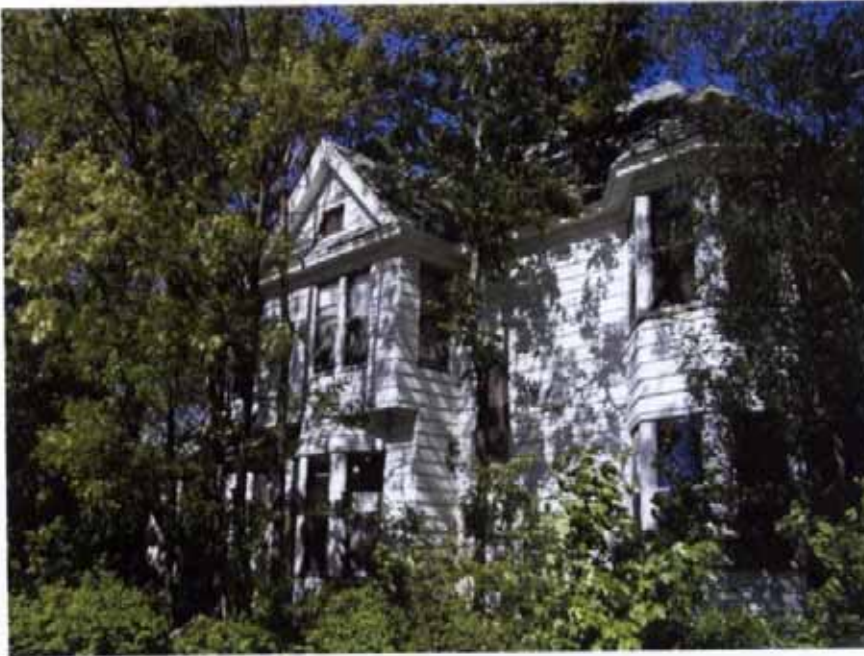
508 West Elm Street. West elevation.
