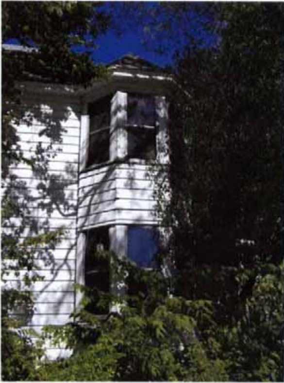
508 West Elm Street. Southwest corner tower.
