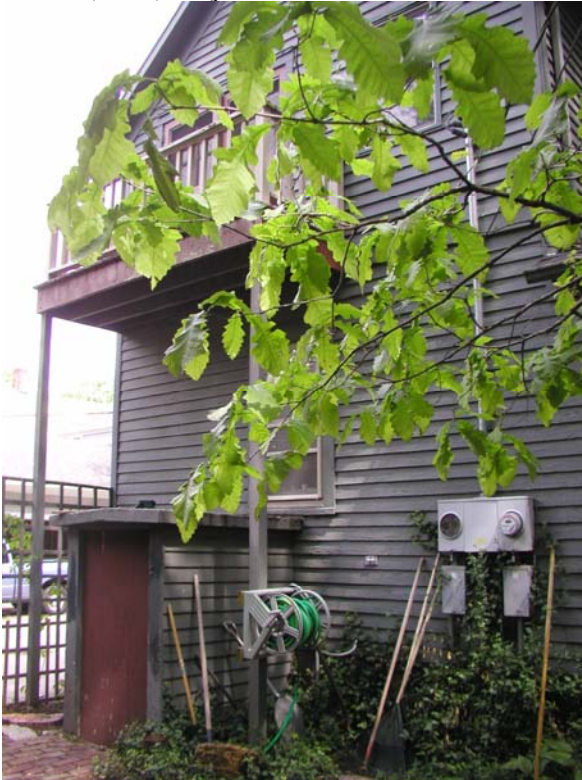
South (Rear) Façade—view from southeast
