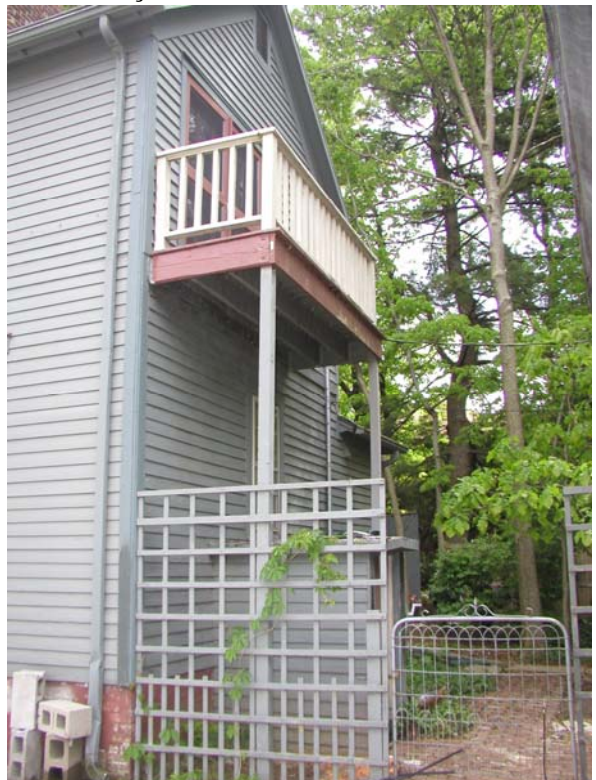
South Façade—view from southwest
