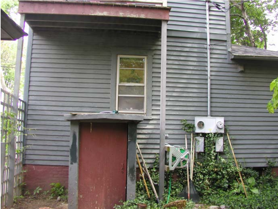
South (Rear) Façade
