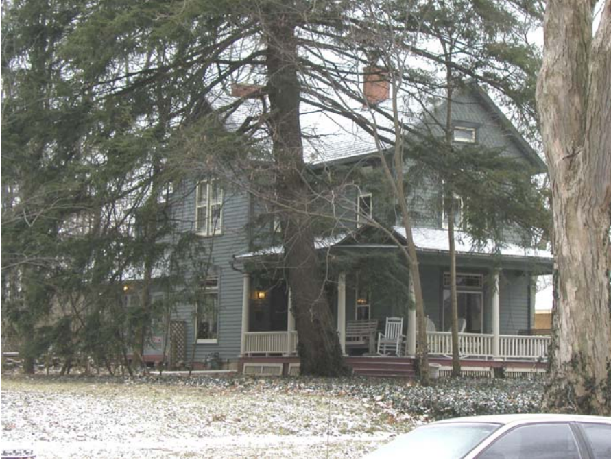
North and East Facades
