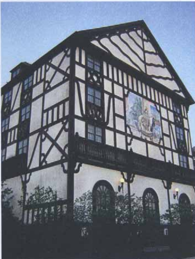
Urbana Lincoln Hotel: 1980's addition, west façade
