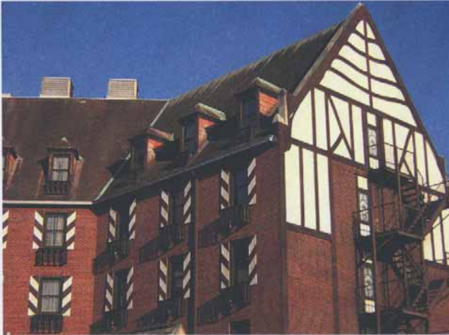
Urbana Lincoln Hotel: Northwest facade
