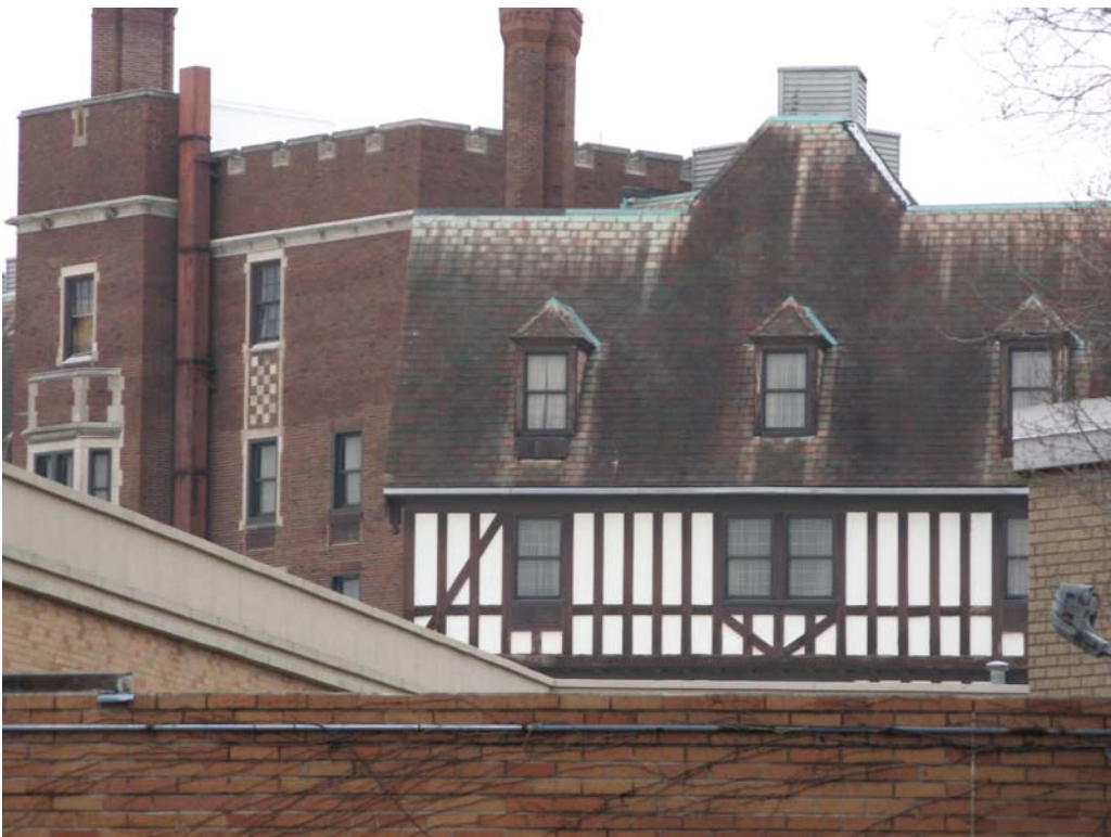
Close up of original 1923 building, east façade
