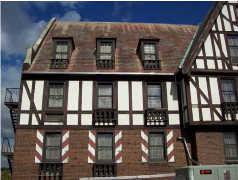
Urbana Lincoln Hotel: South facade
