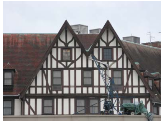
Another view of south facade
