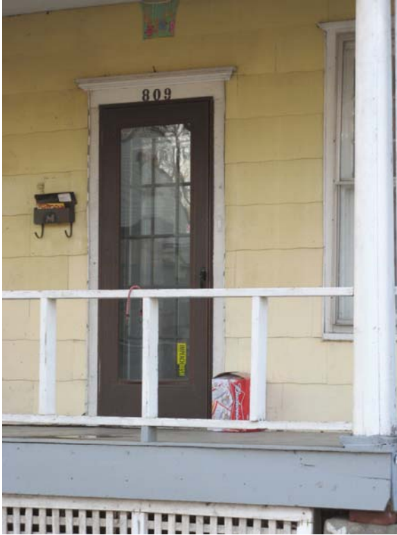
Front door detail
