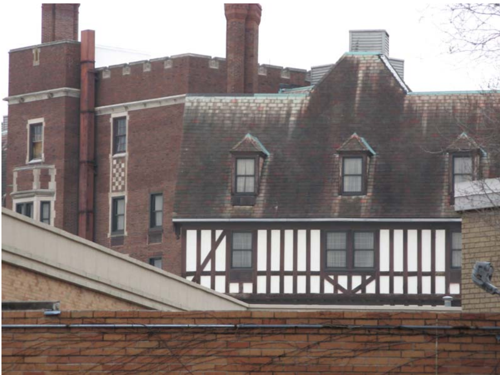
Close up of original 1923 building, east façade
