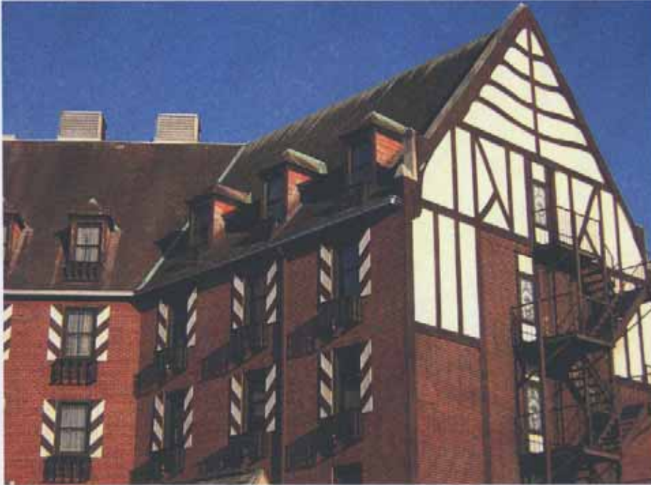
Urbana Lincoln Hotel: Northwest facade
