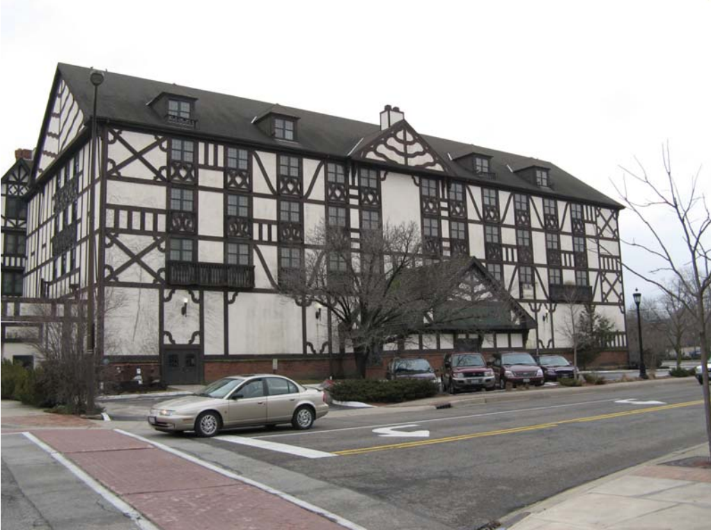
North façade, nearly entirely 1980s addition
