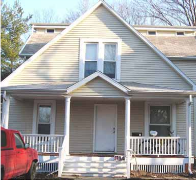
Existing front door
