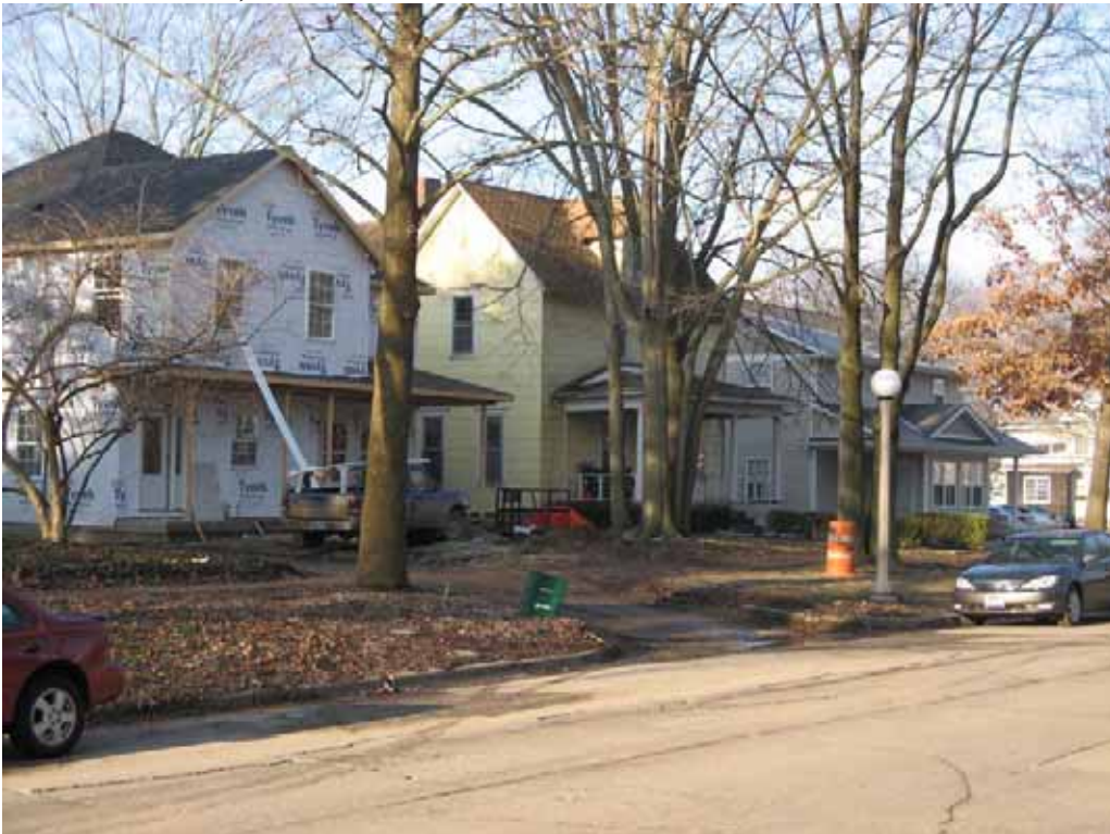
House in context, another view
