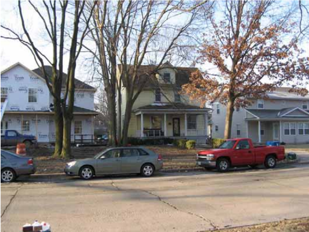
House in context
