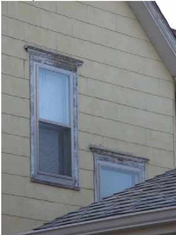
West façade window detail
