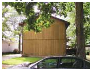
This building is sided with wood, a quality material, but faces sideways instead of facing front. The façade of the building is blank, which can have a negative impact on the neighborhood.
