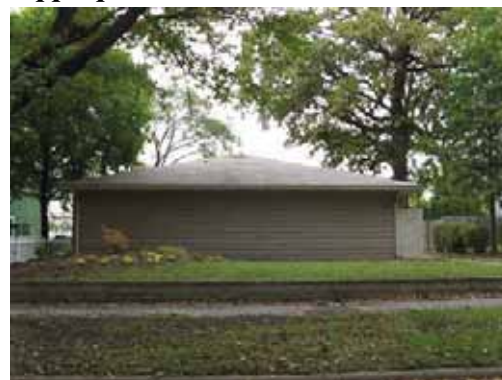
This building has a blank wall facing the street and is not allowed in the design review district.
