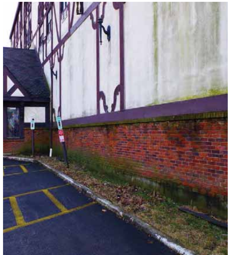
Below: Algae and mold growing on the exterior walls of 201 S. Race. (03/07/2016)
