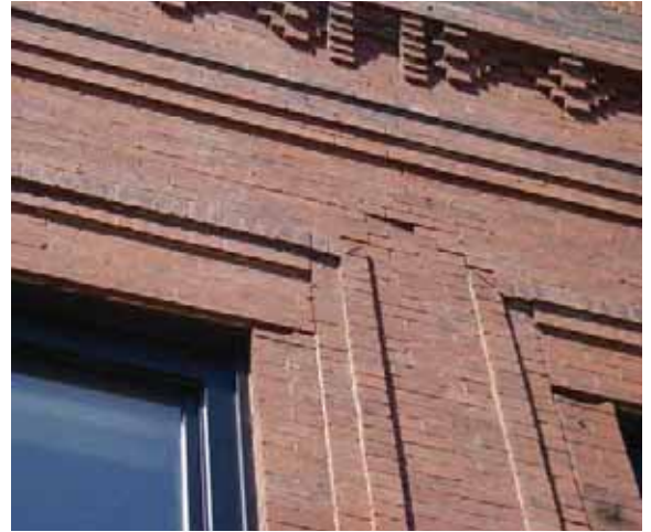
Left & Right: The exterior brick walls at 212 W. Main are exhibit step cracking and deteriorated mortar joints.
