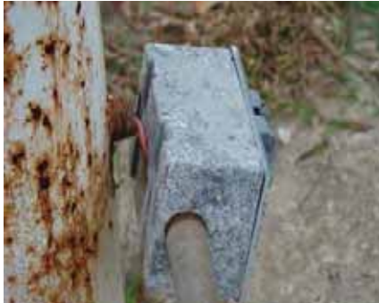
Above and Below: Deteriorated sign post and attached junction box at 207 E. Illinois Street.
