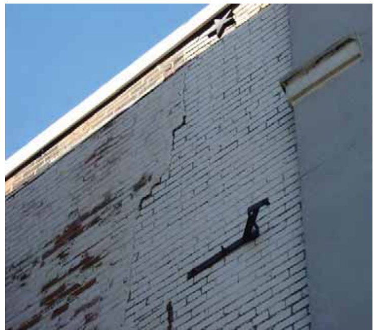
Below: The exterior brick wall at 125 S. Main has step cracking.
