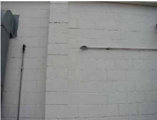
Above: The exterior concrete block wall at 501 S. Vine is in need of tuck-pointing.
