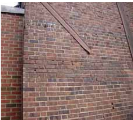
Below: The brick walls at 201 S. Race are in need of tuck-pointing.
