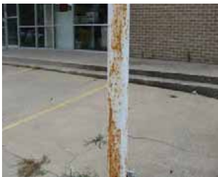
Above and Below: Deteriorated sign post and attached junction box at 207 E. Illinois Street.
