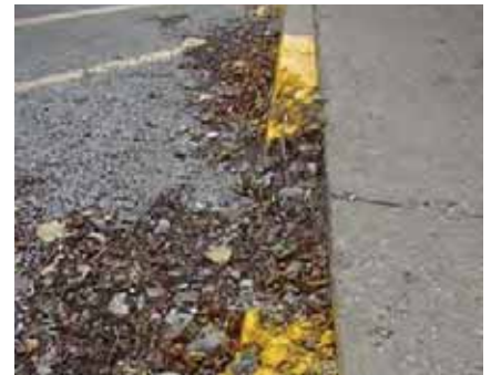
Above: Deteriorated asphalt at 508 S. Vine Street.
