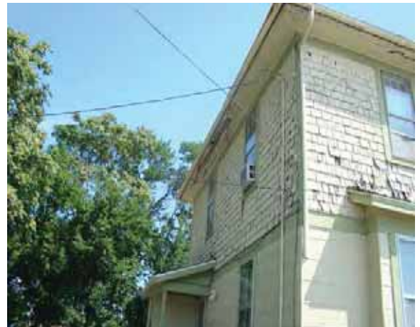
Left & Right: 401 N. Race contains deteriorated wood shake siding and the soffit and fascia has rotted.
