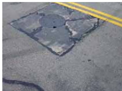
Below: The pavement around this manhole cover on Elm Street is deteriorated.
