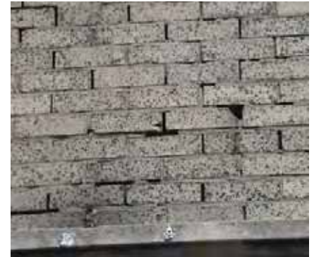
Left: 120 W. Main is in need of tuck-pointing.
