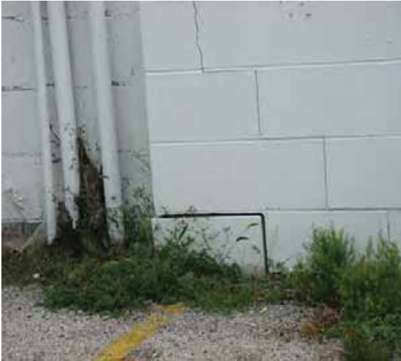
Left: Foundation settlement at 301 E. Main.
