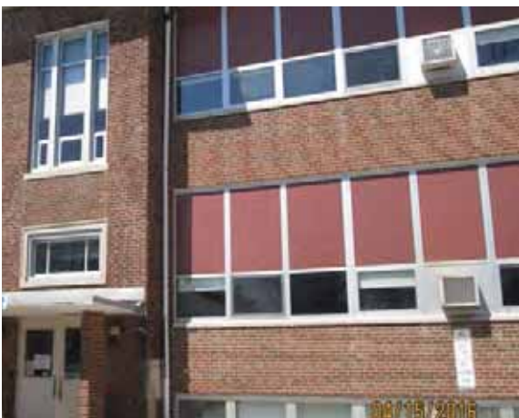
Left & Right: The thermal pane window seals and caulking have failed. (Left picture taken on 04/15/2016. Right picture taken 08/14/2016)
