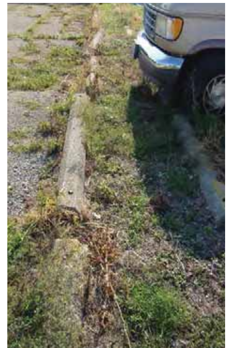
Right: 201 N. Broadway is a deteriorated public parking lot.
