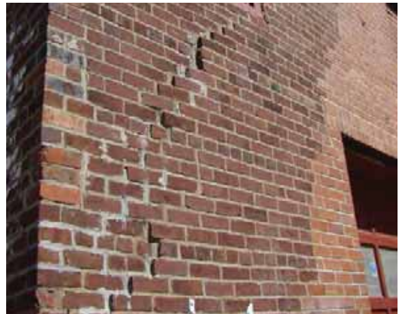
Left & Right: The exterior brick walls at 111 N. Race are sagging and deteriorated.
