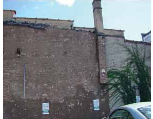
Right: The chimney and exterior brick wall at 201 N. Broadway are deteriorated.
