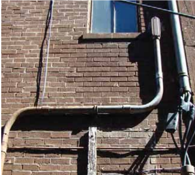
Below & Right: The exterior brick wall at 135 S. Main are deteriorated and in need of tuck-pointing.
