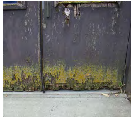
Above: The doorway to one of the halls at 201 S. Race is rotted and deteriorated.
