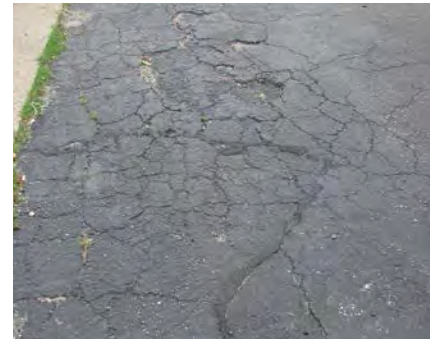
Above: Deteriorated asphalt at 508 S. Vine Street.
