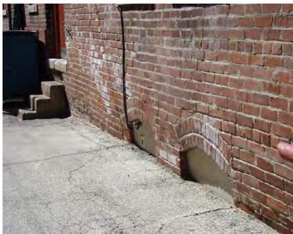
Left & Right: The exterior brick walls at 111 N. Race are sagging and deteriorated.
