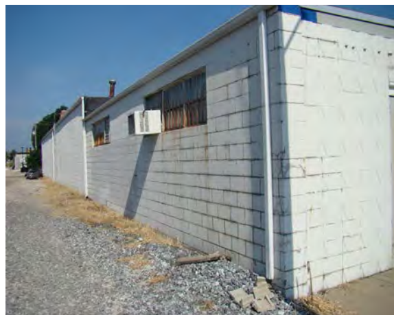
Right: A deteriorated exterior brick wall at 401 N. Broadway.
