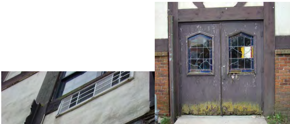
Above: The doorway to one of the halls at 201 S. Race is rotted and deteriorated.
