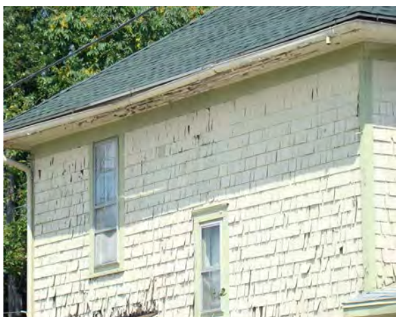
Left & Right: 401 N. Race contains deteriorated wood shake siding and the soffit and fascia has rotted.
