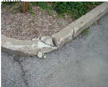
Left, Right, Below, Middle Left, and Middle Right: Deteriorated pavement and damaged curbs and gutters located in the parking lot of 202 S. Broadway Avenue.
