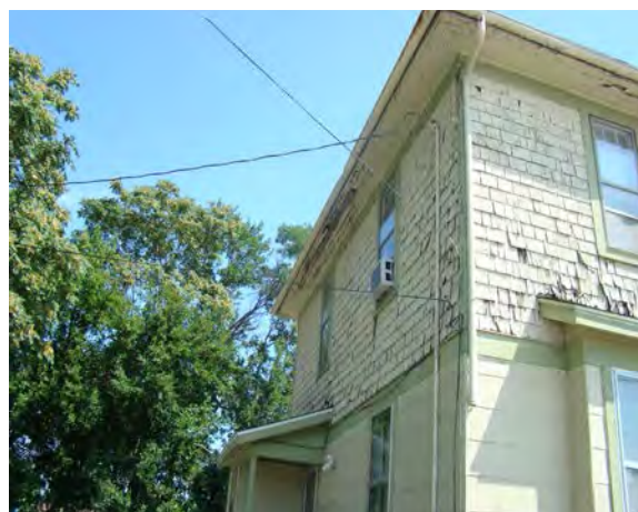
Left & Right: 401 N. Race contains deteriorated wood shake siding and the soffit and fascia has rotted.
