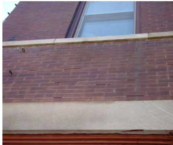
Left: The exterior brick wall at 208 W. Main is in need of tuck-pointing.
