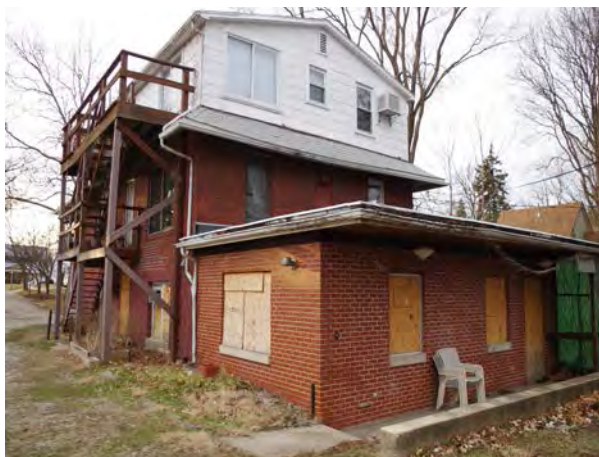
Right: 202 Wood is a deteriorated, boarded up multi-family apartment building with 1 occupied unit. This buildings has deteriorated siding, shingles and gutters. (03/07/2016)
