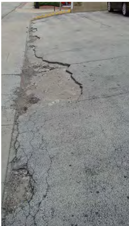
Above: The parking lot for 202 S. Broadway covers the entire lot.
