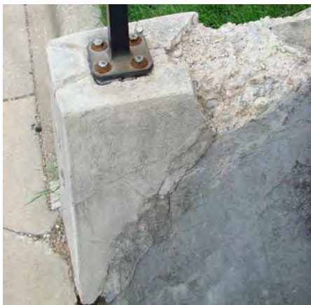
Left, Below, Lower Right, Right, and Above: Deteriorated steps and hand rails located at 202 S. Broadway.
