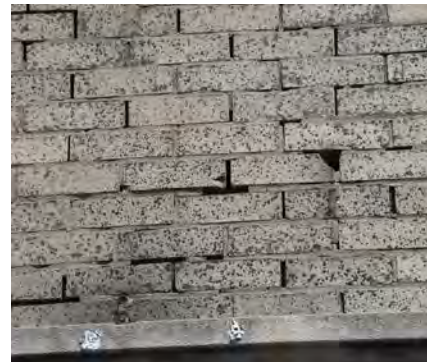
Left: 120 W. Main is in need of tuck-pointing.
