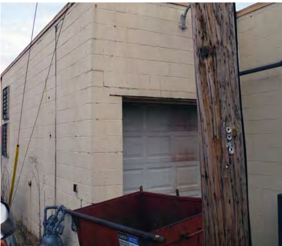
Above: The exterior concrete block wall at 501 S. Vine is in need of tuck-pointing.
