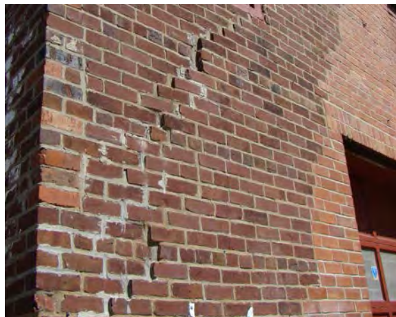
Left & Right: The exterior brick walls at 111 N. Race are sagging and deteriorated.
