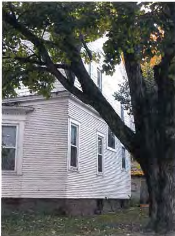
611 West Elm Street: West wall
