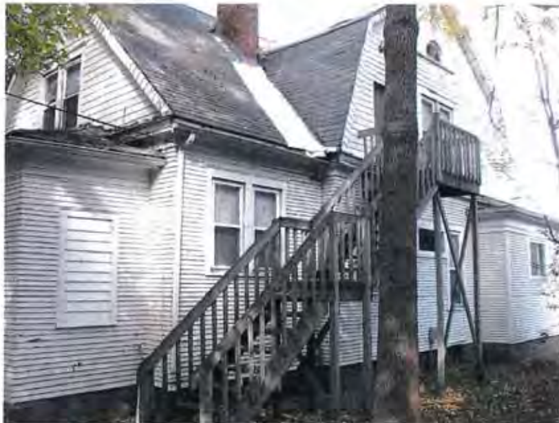
611 West Elm Street: East wall, view from southeast
