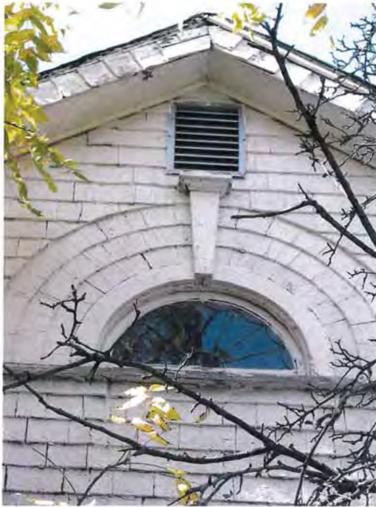
611 West Elm Street: Detail, attic window, east gambrel
