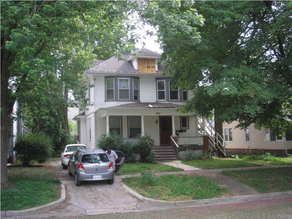
Figure 1. Existing House, front façade
