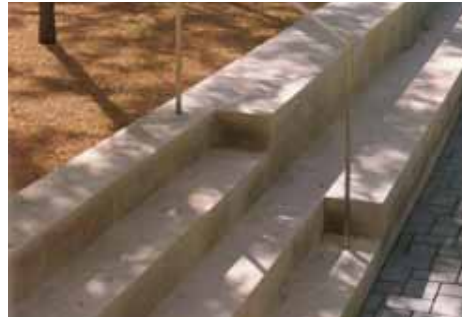
PLANTER WALLS & STEPS
