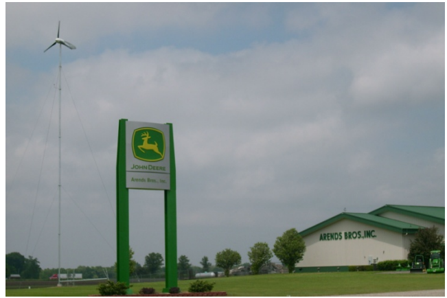
5.0 kW, 21-foot rotor diameter, 115.5-foot system height
