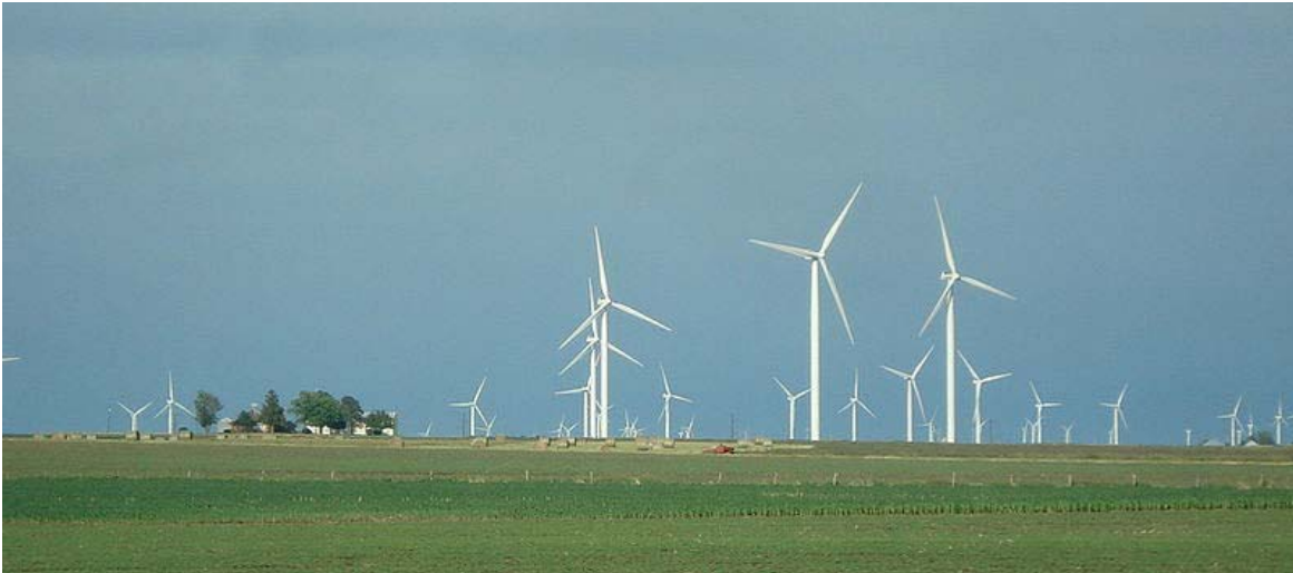
1.65 MW, 269 foot rotor diameter, 214-foot system height
