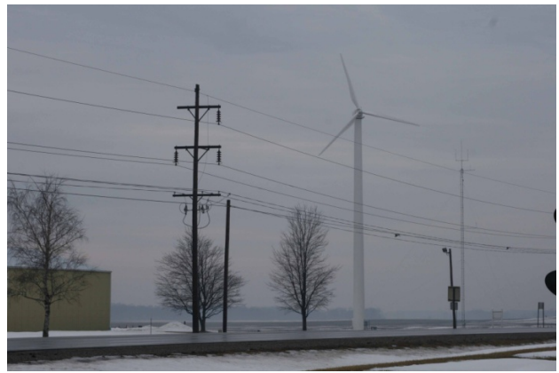
100 kW, 70-foot rotor diameter, 159-foot system height
