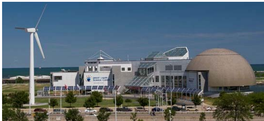
225 kW, 88.6 foot rotor diameter, 150 foot system height
