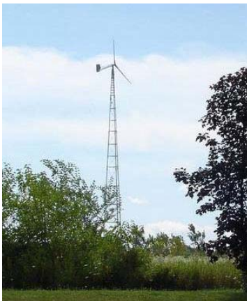
20 kW, 100-foot system height
