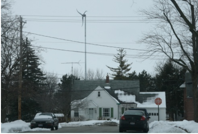
2.4 kW, 12-foot rotor diameter, 60 foot system height
