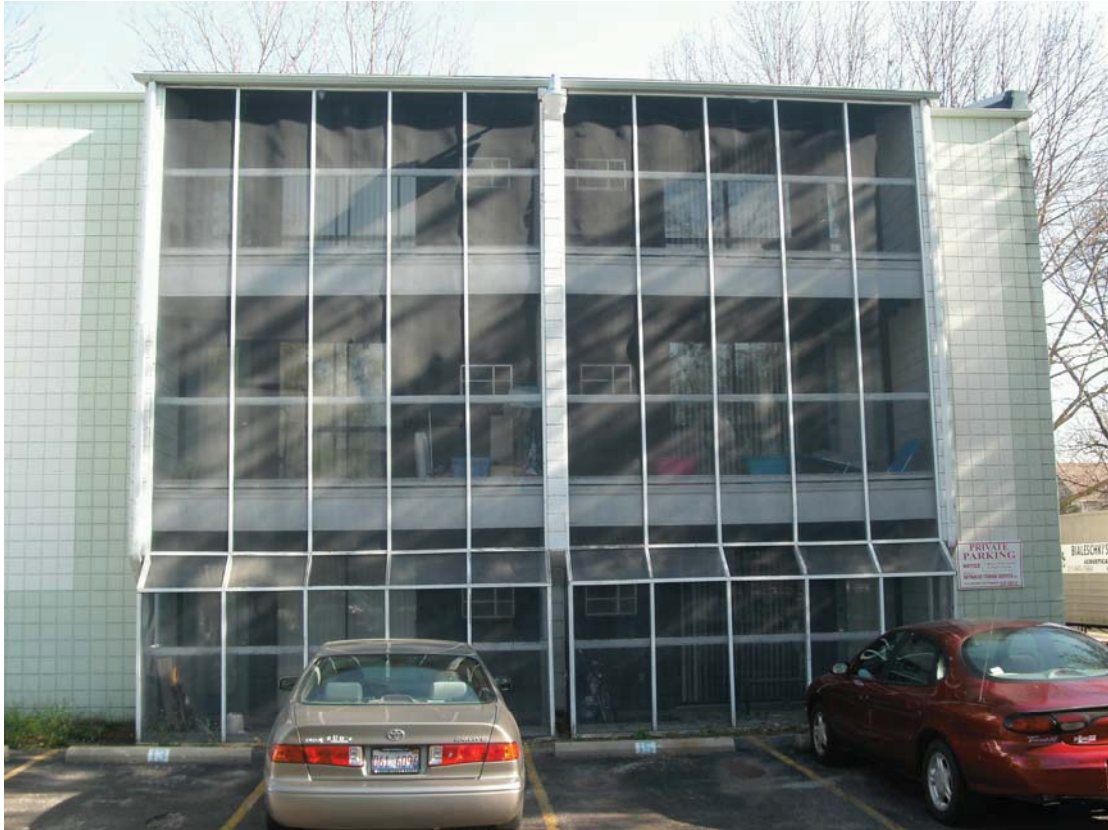
BUSEY COURT APARTMENTS – TYPICAL EXISTING BALCONIES
