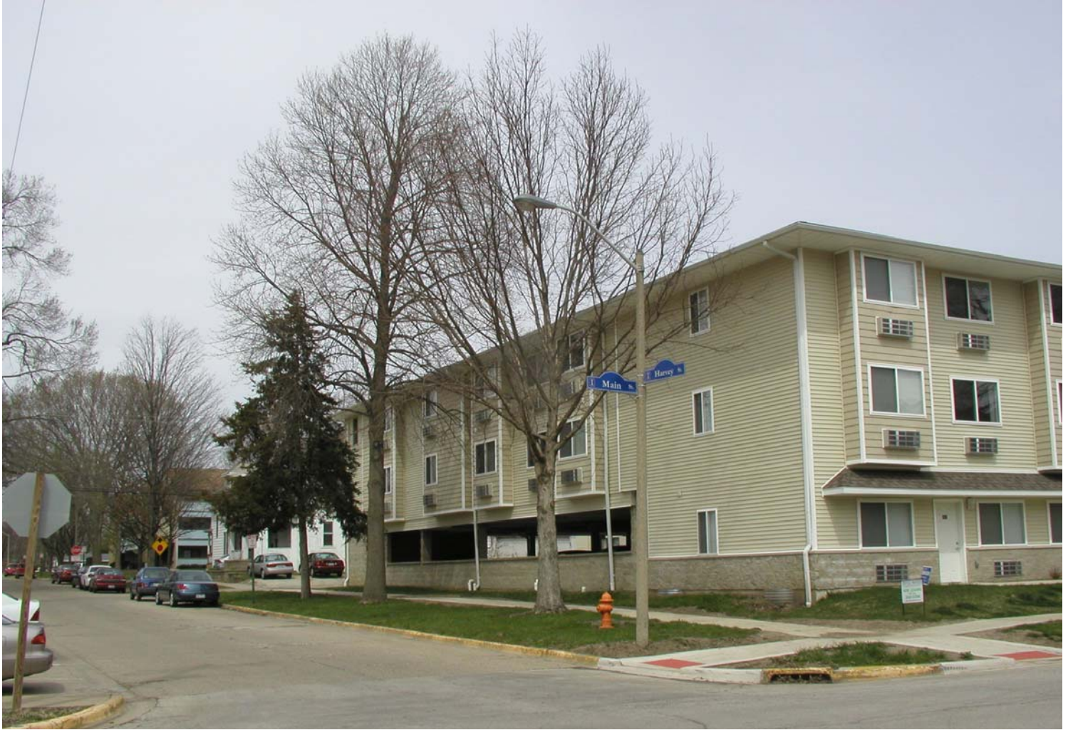
Figure 3. View of 1010 West Main, looking north along Harvey Street
